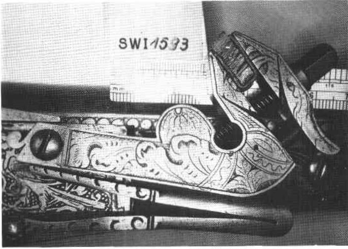
The replaced cock on the pistol. *It should be noted that we do not undertake the reconversion of former flint locks. This is a matter of principal.*
