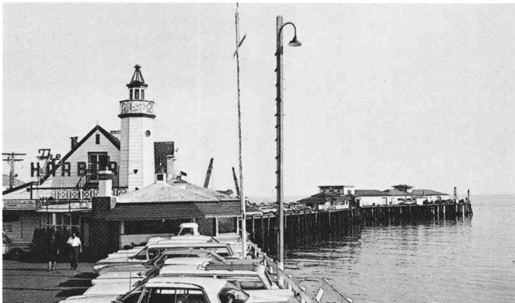
There's always room for expansion at Santa Barbara.
