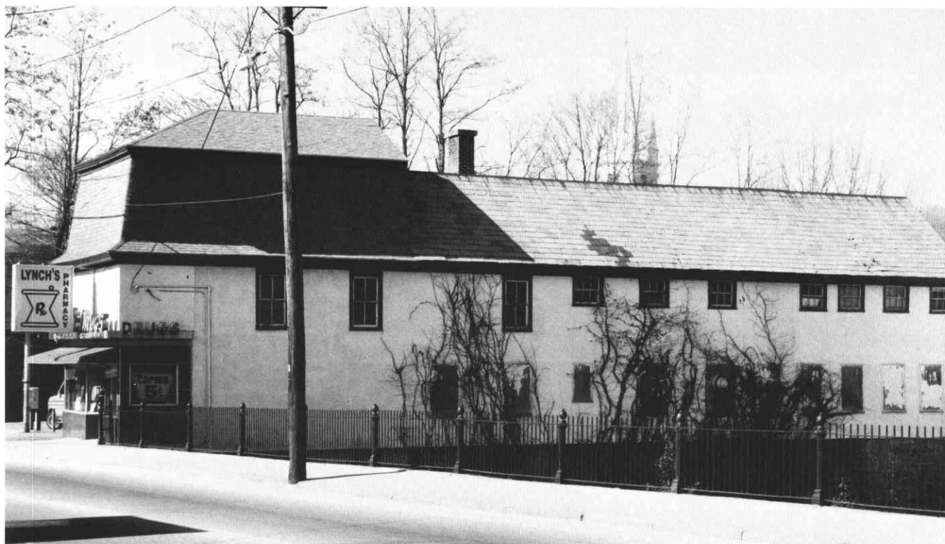
RIFLE SHOP OF THE BAY STATE ARMS CO. The original two-story section was built as a grist mill in 1777; a 30 foot mansard roof addition was completed in 1885. Steam heated and gas lighted, the shop was adjacent to the Mumford River, which provided power for the machinery. Of an estimated shop force of 8-10 workmen, eight families followed the machinery to relocate in Norwich, Connecticut, in February 1887.
