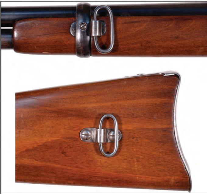
Figure 3. Side swivels added by French armory.
