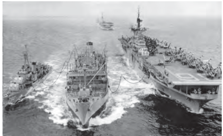
Navy ships refueling underway, after line throwing guns to get shot lines across to pass the heavier lines and hoses. U.S. Navy photo.
