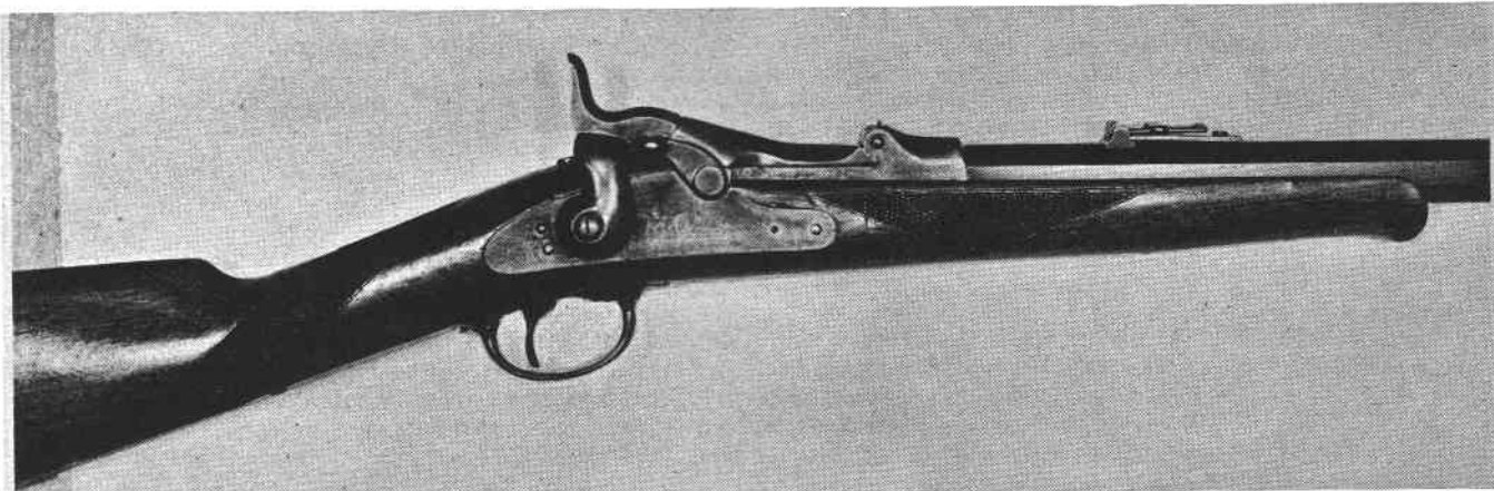
The "So Called" Marksman Rifle, which was in reality a rifle assembled from condemned parts by the Hartley & Graham Co.
