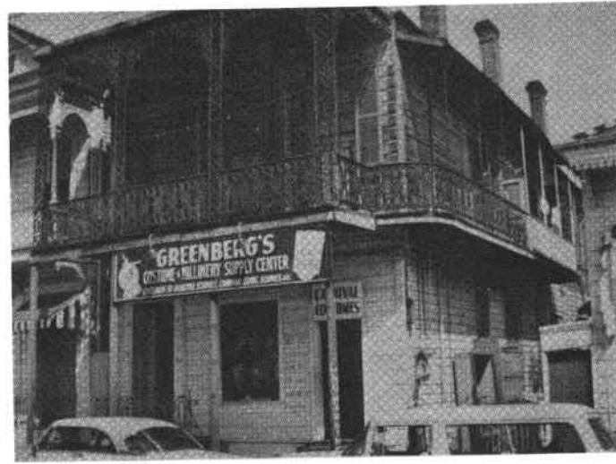
NUMBER 203 PAMPART STREET IS NOW 912 RAMPART STREET. THIS WAS THE 1860 RESIDENCE OF DR. LE MAT. Photo by Charles L. Durour, New Orleans, Louisiana.
