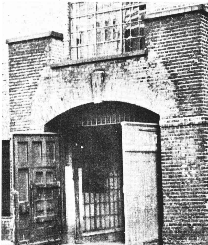
Figure 1: Colt factory on the Thames bank near Vauxhall Bridge.
