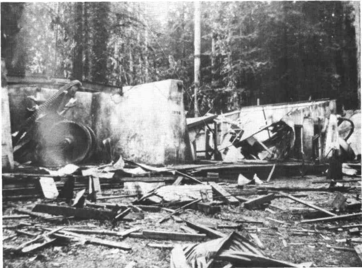
Damage to the wheelhouse after the explosion of 1898.
