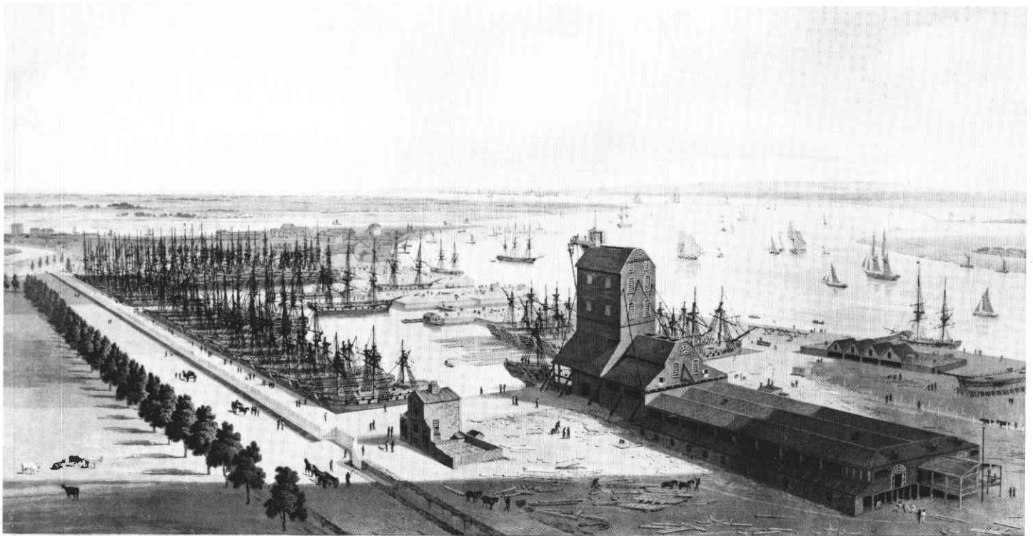
Brunswick Dock on the Thames at Blackwall The middle house was erected from the designs of the celebrated architect Adam (after) King & was built intended for the accommodation & purchase of the ships of the East India Company. The whole operation which relates about masts was in detail seen from the East India Company's office of which he reports of building them in the Island Black India village in the other one was made in another style. This part of masts were not built on the 17th of March 1790 in the Dock, who served in the capacity of carpenter on the 17th 1790. To Adam King & John Price in and was purchased approved by Sir Andrew Boscawen, General, Admiral.
