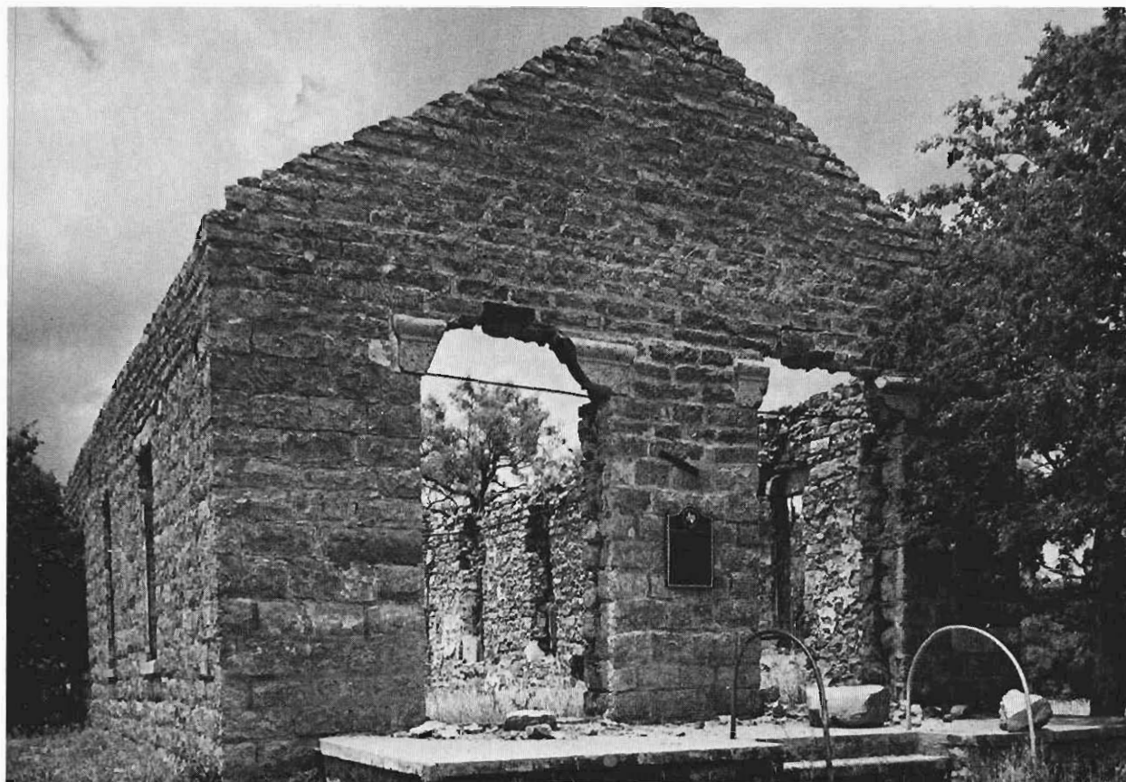
Masonic Temple remains. The only structure standing in The Flat at Fort Griffin today.
