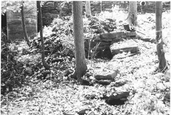
Closer to the dam and some of the mill wall.
