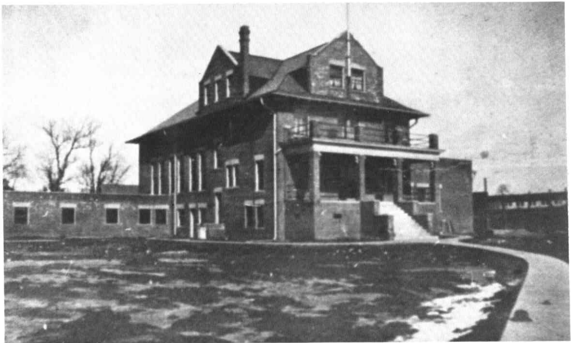
The West Allis Shooting Park headquarters building.
