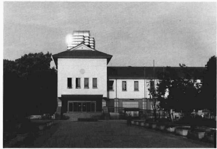
... and the front of the renovated building.
