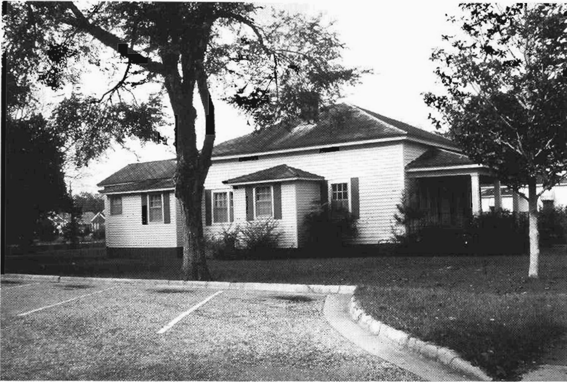
Figure 6. Operative's quarters built by the Ordnance Department on King Street in 1865 as they look today. "Operatives" were supervisors and managers.
