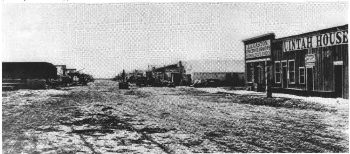
Figure 10. A view looking toward the other end of Corinne's Main Street. The familiar rifle-sign of Freund & Bro. can be seen over the street in the left background. (Photo by William Henry Jackson)
