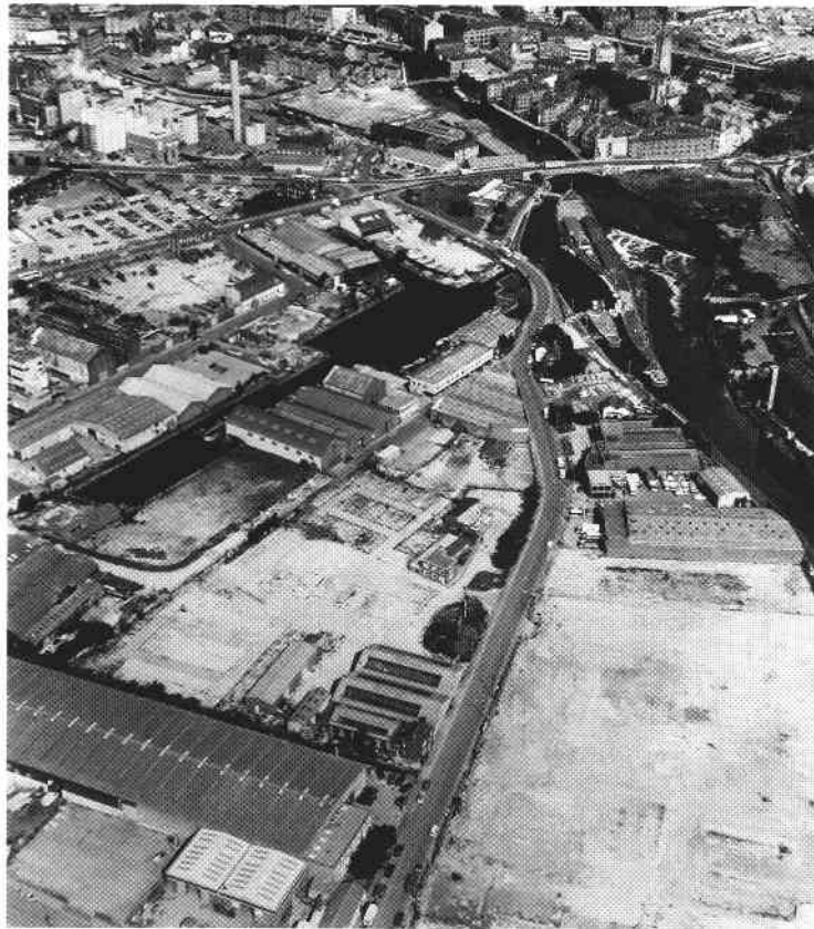
Figure 6. The site at Clarence Dock before building commenced. Photograph courtesy of West Yorkshire Police Photographic Department.
