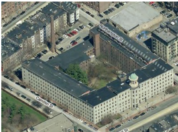
Figure 7. Aerial view of the Chickering Building today.
