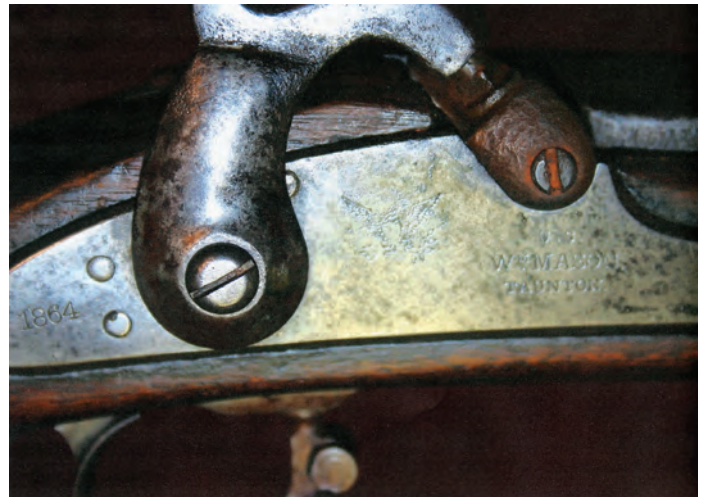
Figure 21. Standard 1864 lockplate markings. (Author's Collection)
