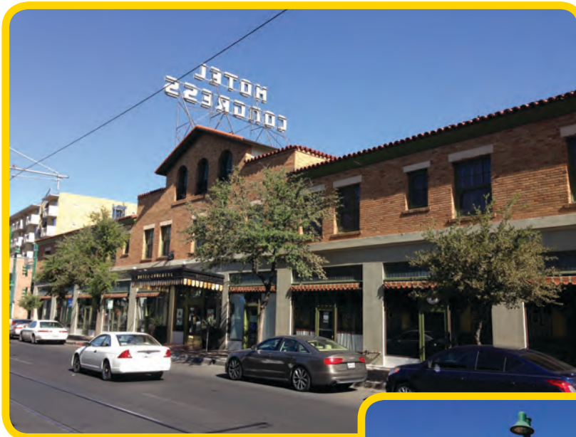
The Hotel Congress as it appears today. Notice how the Hotel is only two stories tall today, after the third story was destroyed in the fire in 1934. (Photo Tracie Hill)
