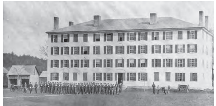
The Norwich University South Barracks in Norwich Vermont during the late 1850's
