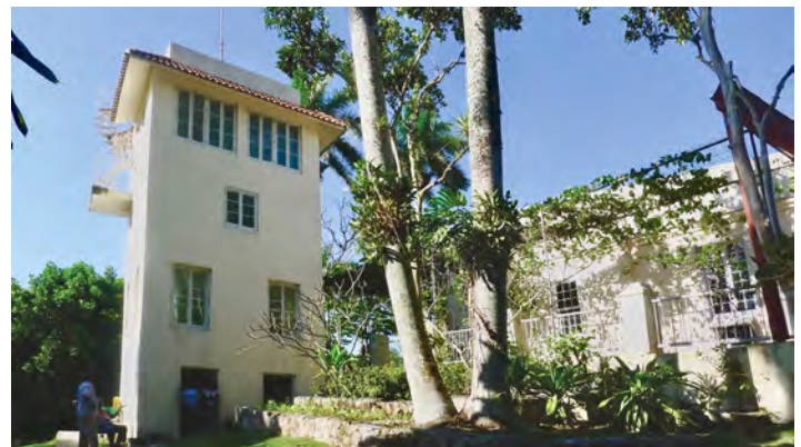
Figure 2 - The tower side of the Finca Vigía, an Italianate villa built in 1886 and bought by Hemingway in 1940 for $12,500. With private help from the US, Cuba has been able to refurbish and stabilize the house, but in a tropical climate this is an ongoing campaign. The Finca contains Hemingway's library of 9,000 books as well as thousands of letters, manuscripts and photographs and most of Ernest and Mary's furnishings and belongings. (Steve Helsley)
