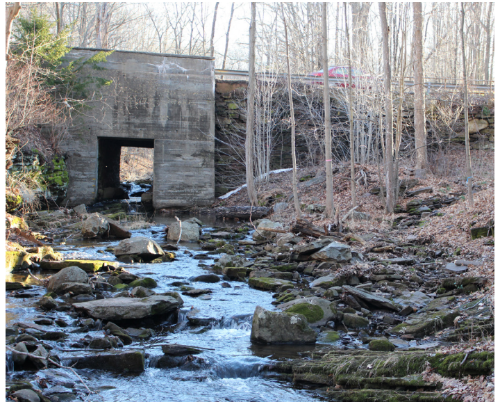
Figure 6. Spruce Brook mill dam.
