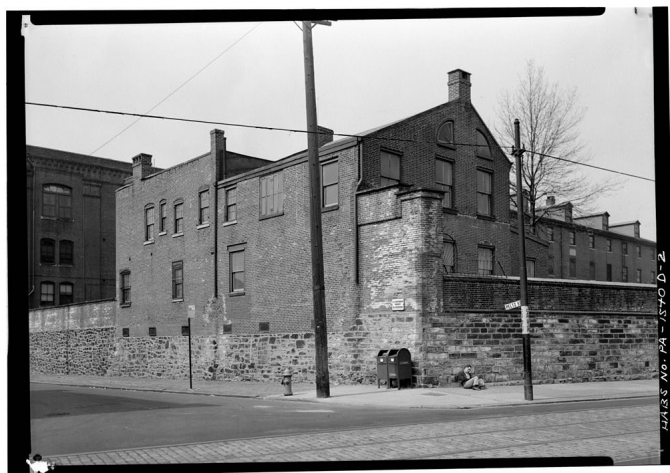
Figure 21. One of the original buildings of Schuylkill Arsenal, Philadelphia completed in 1801.
