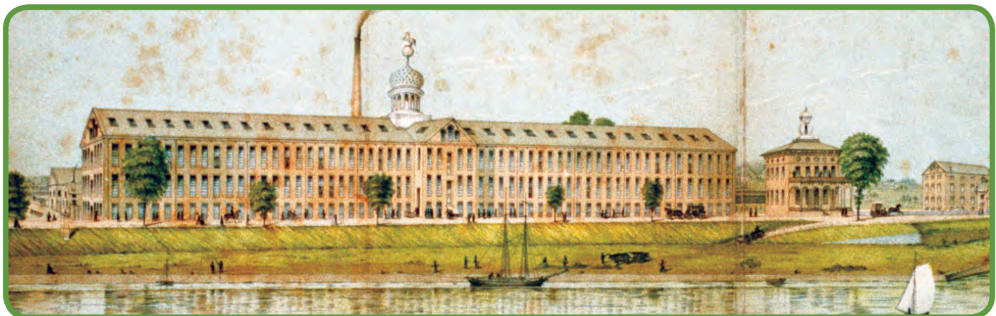
The Colt 2nd factory, circa 1855, along side the Connecticut River on a 260 acre site.
