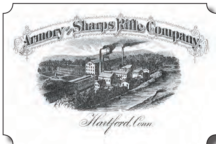
This is the Sharps Rifle Manufacturing Company's letterhead, depicting its factory at 436 Capital Avenue.
