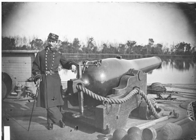
Figure 3. A IX-inch Dahlgren shell gun.
