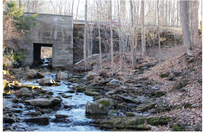
Figure 6. Spruce Brook mill dam.
