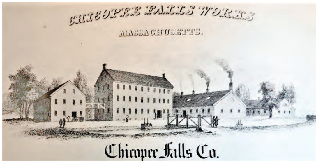
Figure 4. Image of the Works of the Chicopee Falls Company from the company's trade card about 1838 (Photograph by Peter Buxton). The buildings shown, from the left are the saw house, the gun shop, the forge and the furnace. The foundry is to the right and on the near side of the canal shown running in front of these buildings (not shown).
