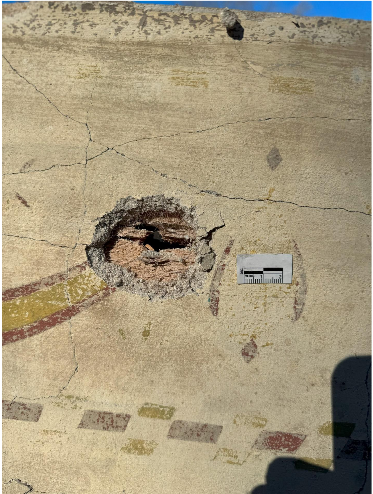
Figure 27. Detail of the exit hole in the plaster of Wall Section 3.
