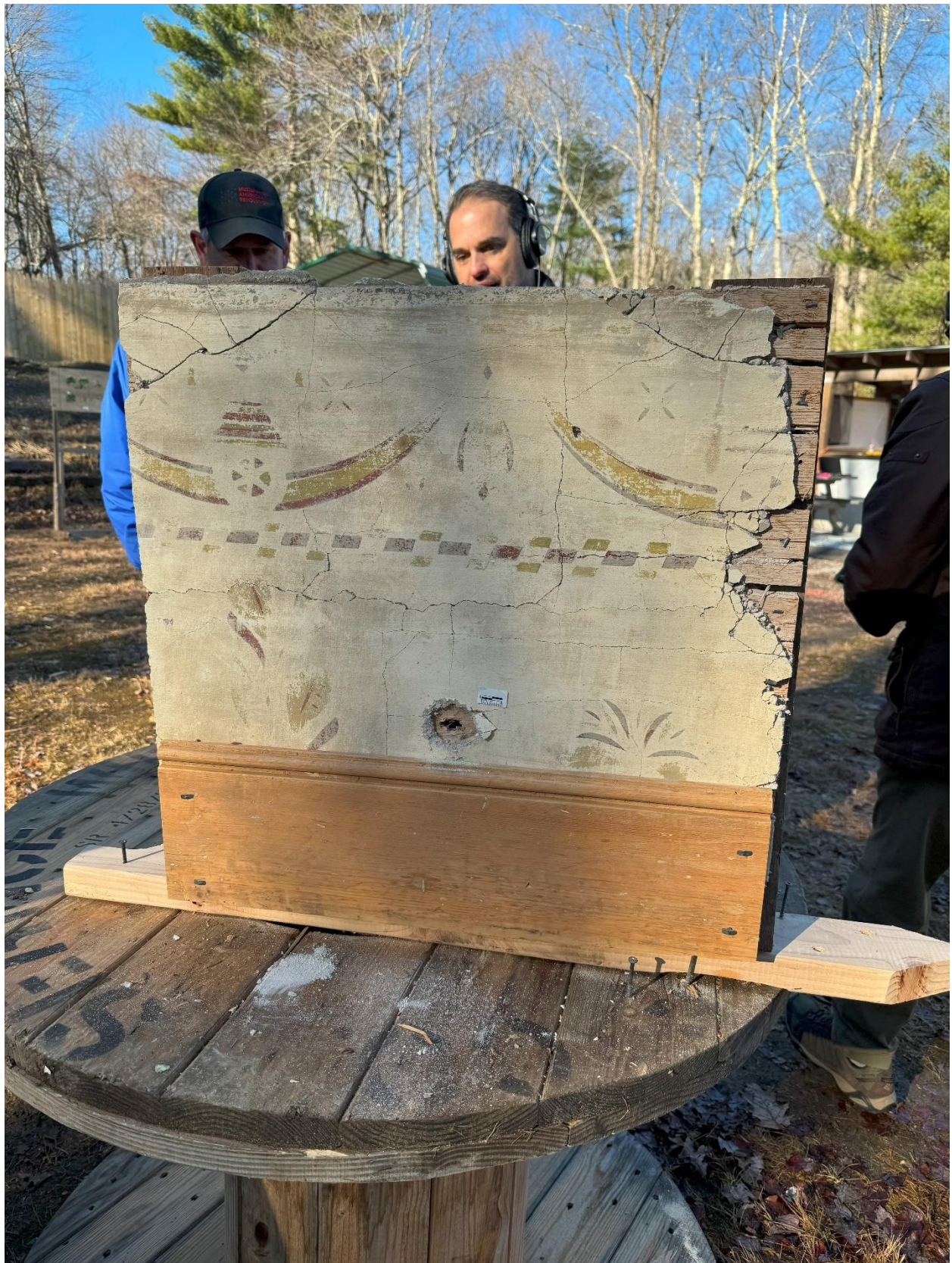
Figure 26. Exit hole around the plaster of Wall Section 3, Shot 1.
