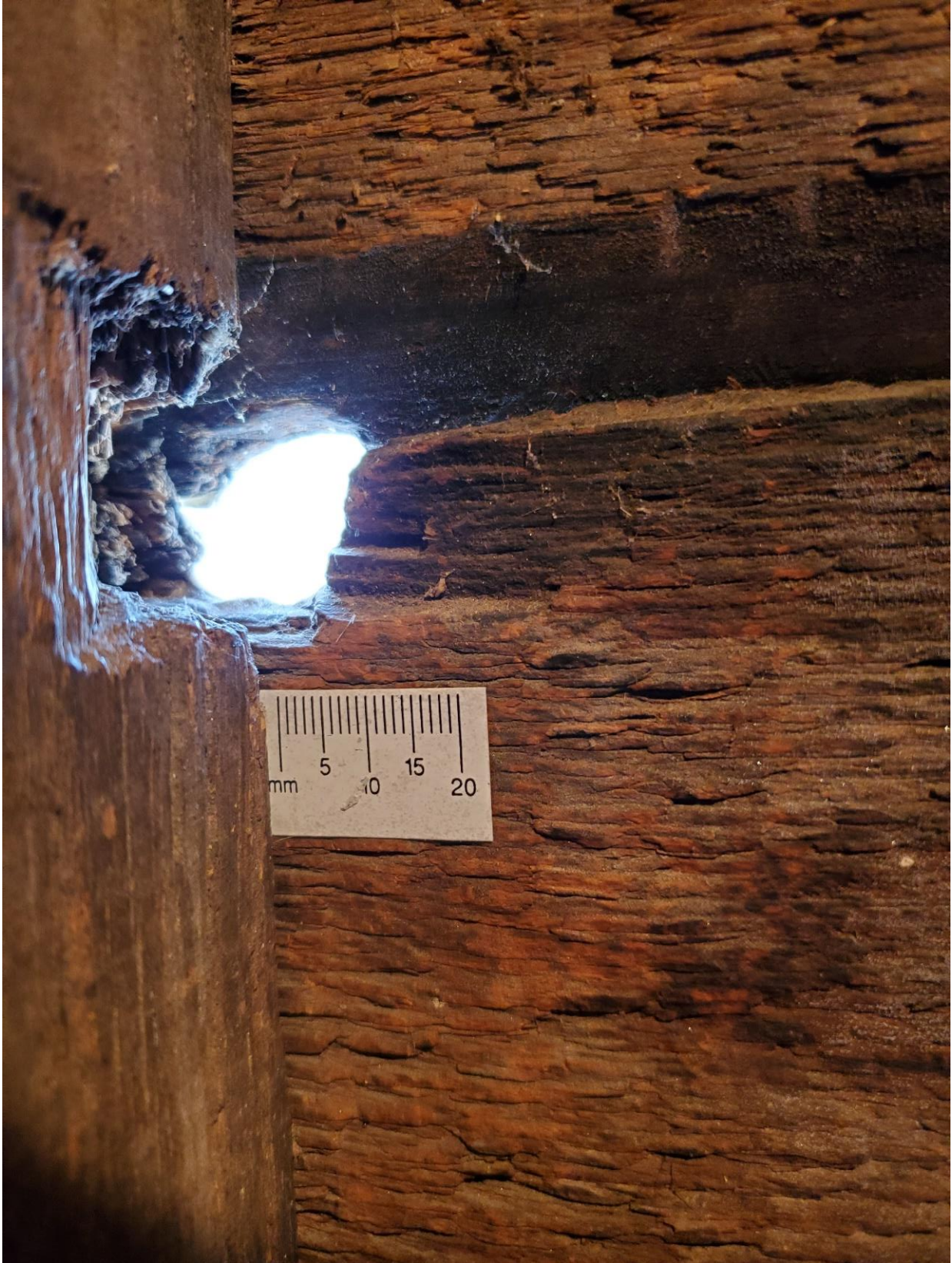
Figure 19. The bullet struck a sheathing feather edge joint on the Elisha Jones shed interior wall.
