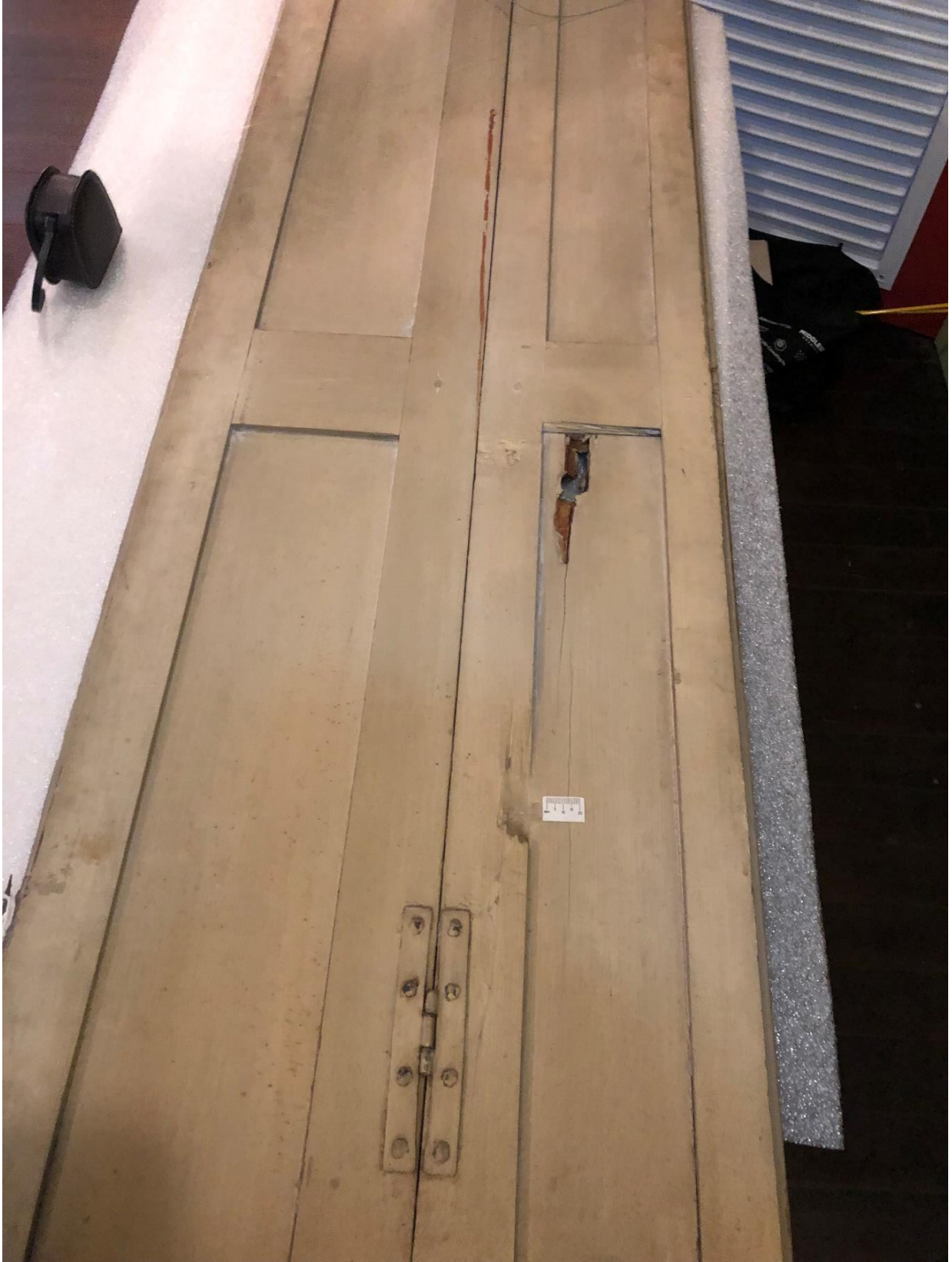
Figure 28. Bullet-struck interior shutters removed from their original context and now part of the Arlington Historical Society collection.
