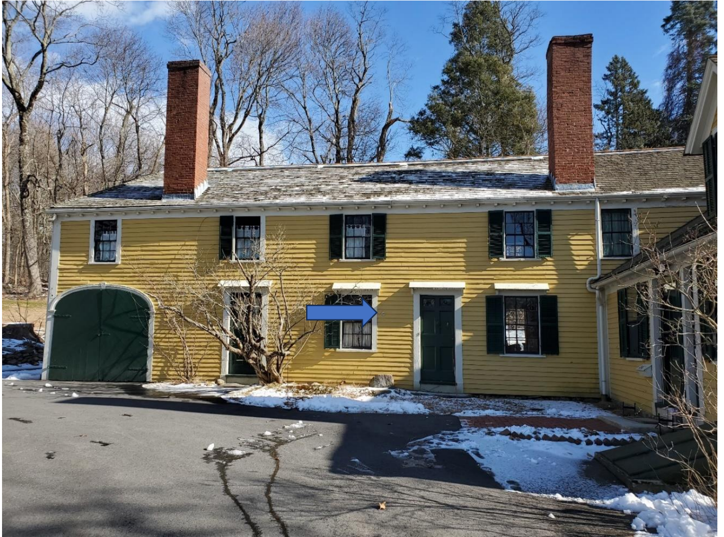
Figure 18. The Elisha Jones shed currently attached to the original house. The bullet strike is to the immediate right of the window in the center of the image.
