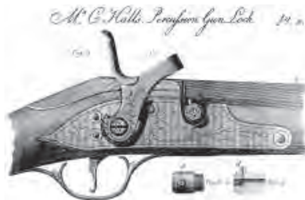
A152 Fig. 11.11 Collinson Hall's Patch Lock was announced to the public in the 1817 report of the Royal Society of the Arts. He described the "cylindrical plug" screwed into the barrel and the "pin or nipple" protruding from it at right angles thus creating new words for arms historians.
