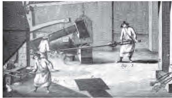
A761 Fig. 13.7 A water-powered hammer (lower right corner) being used to shape the beat the slag from wrought iron illustrated by Georgius Agricola in De Re Metallica , 1556.
