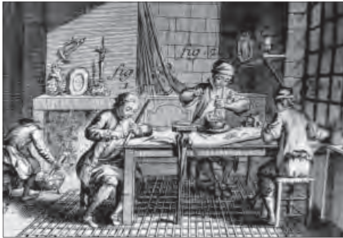
A305 Fig. 13.28 A view of the interior of the workshop of a Ciseleur et Damasqu shoreur (engraver and [gold] damascener) from the Diderot Encyclopédie c.1760. On the left, an engraver working on a gun barrel with a group of barrels and two sporting guns resting in the corner.
